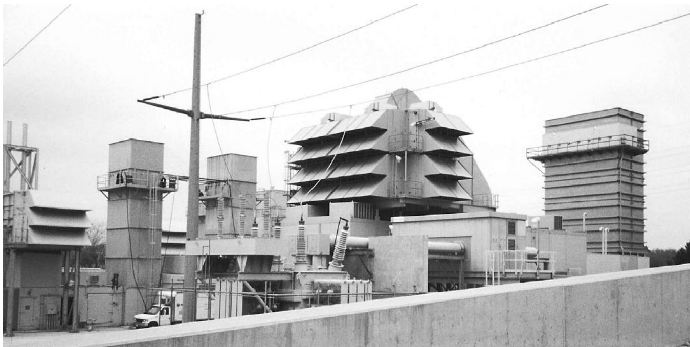
Fig. 1— An aero-derivative combustion turbine (unit with dual stacks) rated at 50 MW next to an industrial combustion turbine rated at 120 MW. Hooded assemblies are combustion air inlets. Vertical rectangular stack assemblies are turbine exhaust silencers venting to atmosphere.
